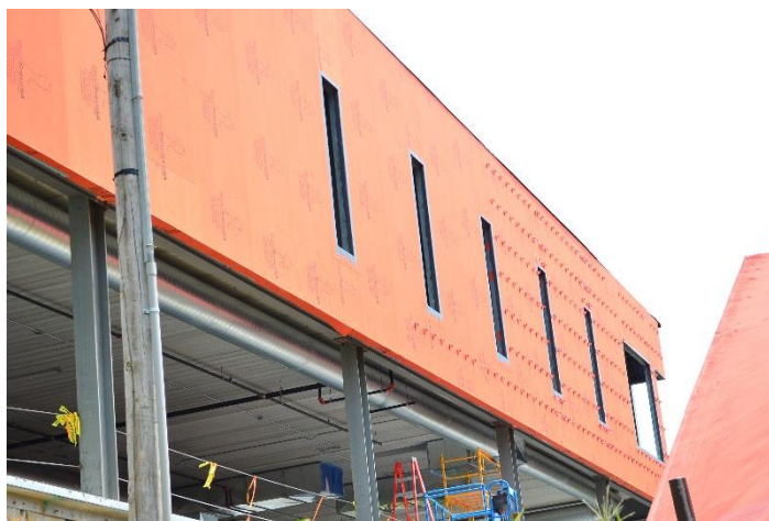
WrapShield SA Self-Adhered contributed to the building's sustainability because of it being 100% recyclable, having zero VOC's and not requiring primer.
