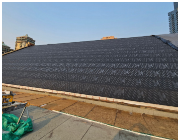
Standing Seam Metal Roof
